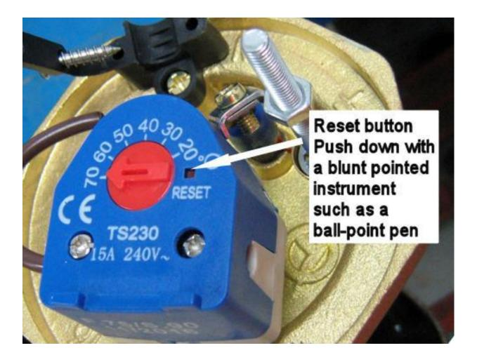
If the thermostat has tripped then the button will be flush with the top of the plastic housing. We recommend the use of a ball point pen or similar tool to push it down (small screwdrivers are usually too big to fit through the hole) and when it resets it will go down with a noticeable click. Once it is reset the button will be about 1.5mm below the surface of the housing.
